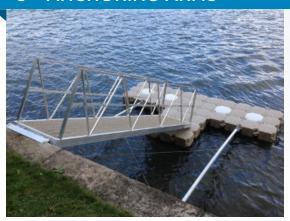
The anchoring arms technique is a lesser employed option but can be proven necessary in some cases. Generally speaking, the anchoring of a floating dock using this technique will impose a few basic restrictions:
